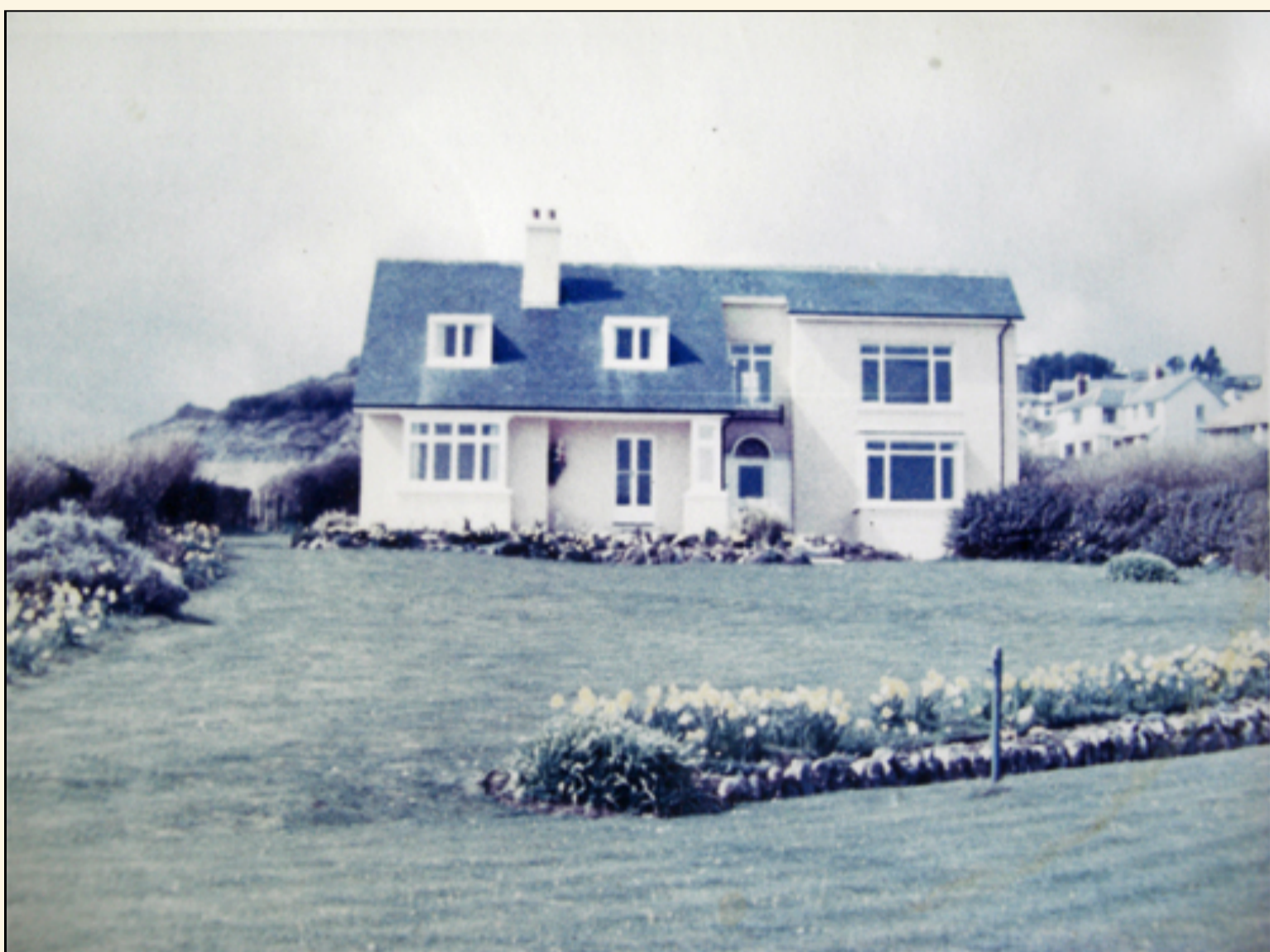
Thalatta not long after the extension was added in 1964, notice the lower windows on the 1922 building has more panes than today.
