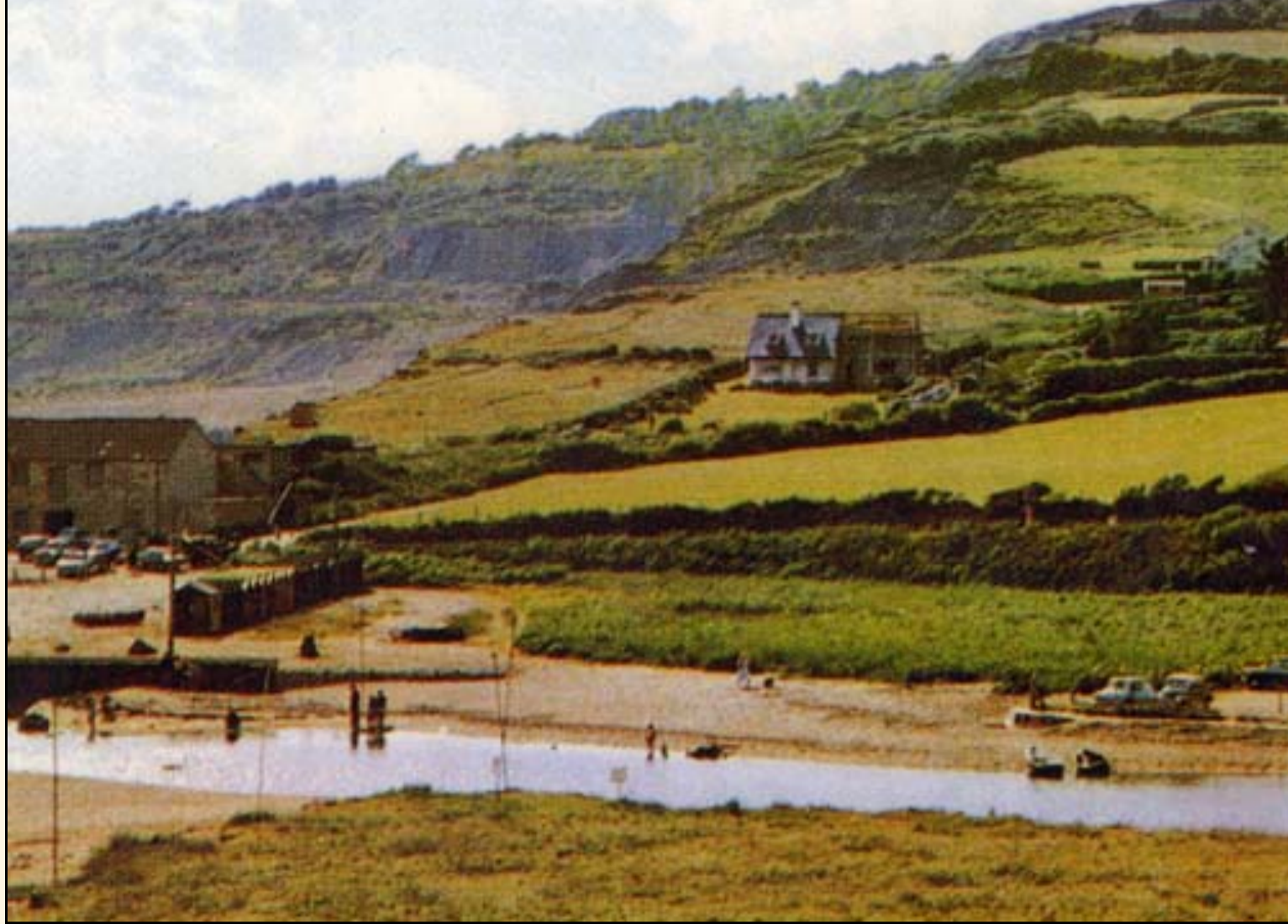
Thalatta with the extension being in the process of being added in 1964,
